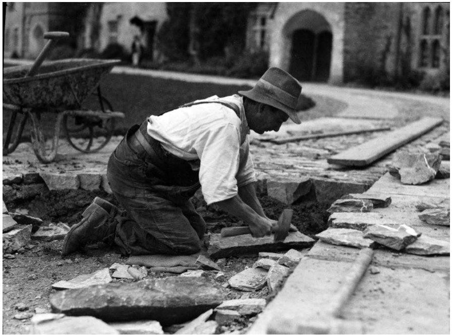
Laying Stone Path in Courtyard, Early 1930's.
